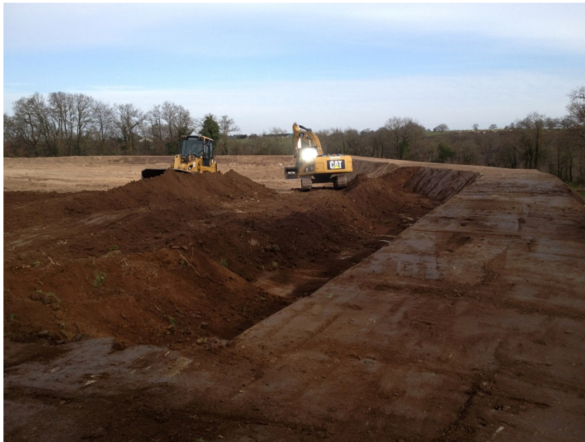
Figure 4: Conception de digues. (Crédit photo Idra)
